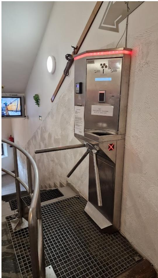
Tripod turnstile with integrated coin machine and bank terminal for quick and convenient access to toilet or other facilities. Integrated anti panic function and free exit. The turnstile cabinet is made of brushed stainless steel sheet metal with a thickness of 1,5 mm, rotating arms of stainless steel tubes, diameter 40 mm, length 500 mm.
